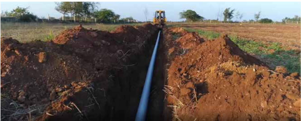
Aquasafe pipes being installed at one of the farms of Halvad, Gujarat.
