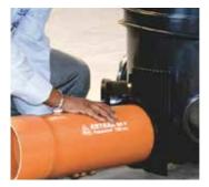
9 FIX PIPE IN INLET (\*DRAINMASTER,FOAMCORE, D-REX PIPE)
